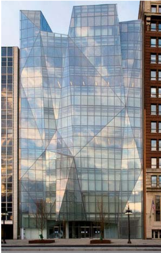
FIGURE 2: SPERTUS FAÇADE (EAST FACING)
